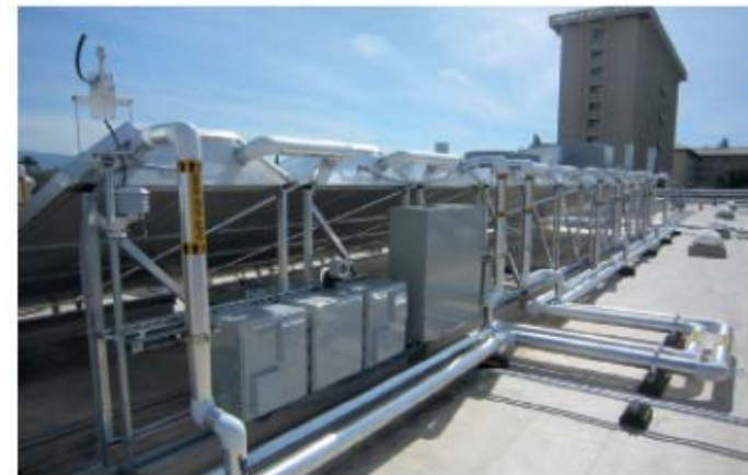
Rear view of MCT collectors & piping at the Benson Center
