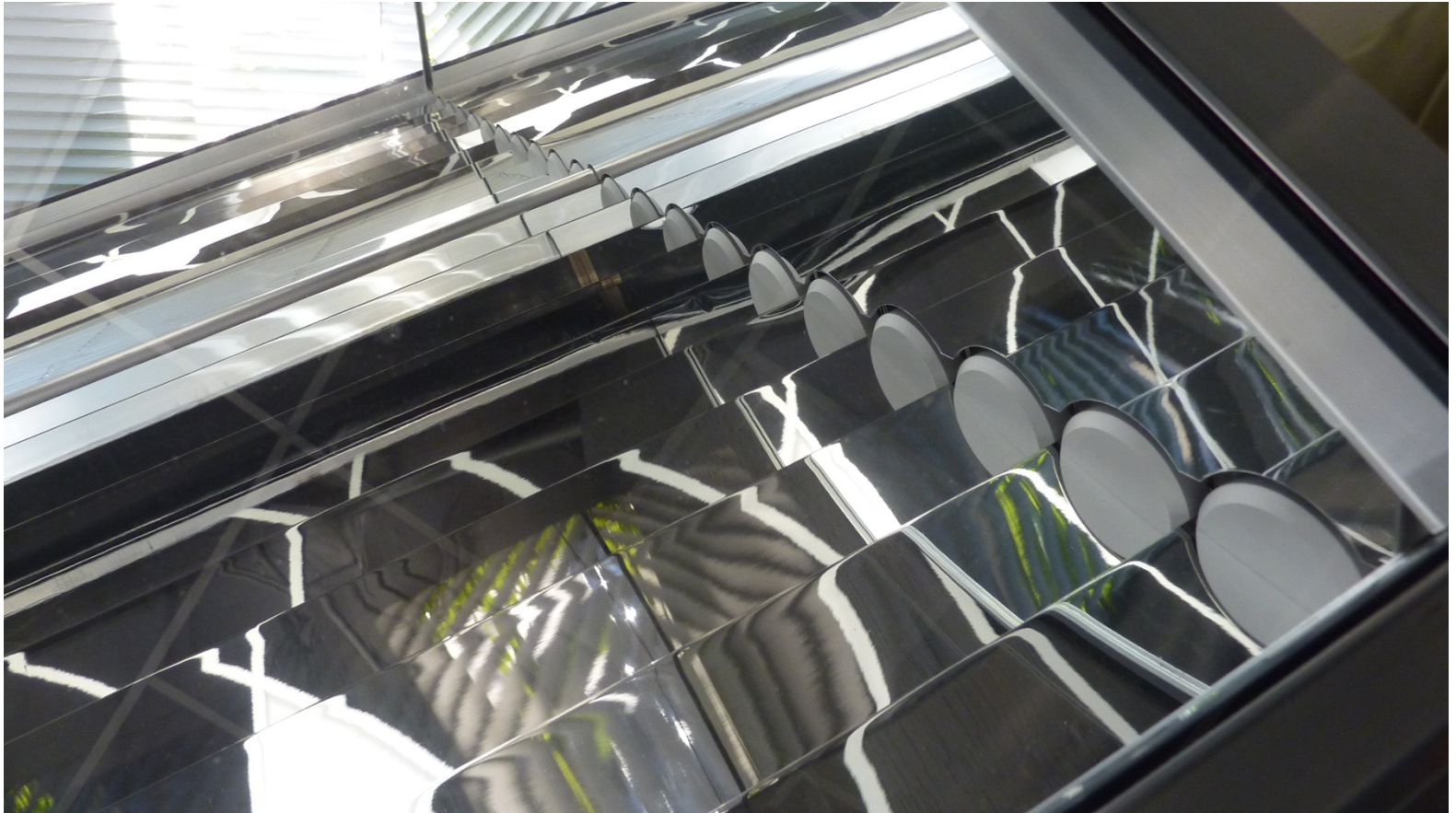
Series of Angled Fresnel Mirrors
