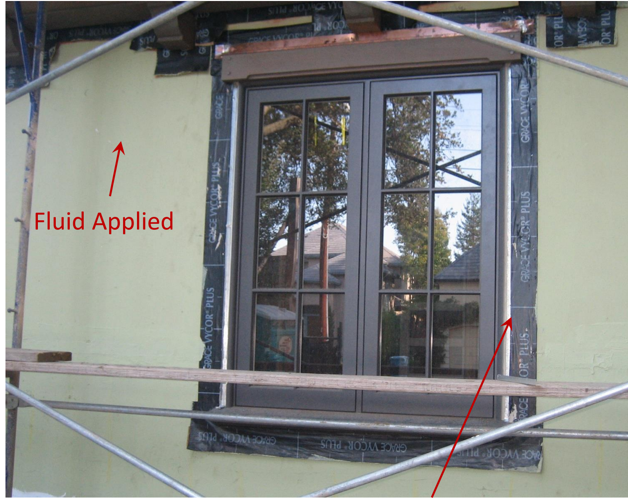
Window sealed with Flexible Flashings
