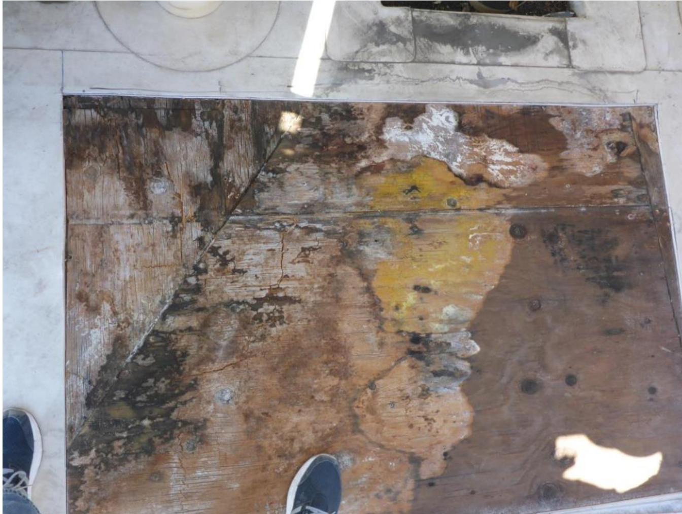
Destructive Test Cut #7b, Damage Level 900 (condensation related)
