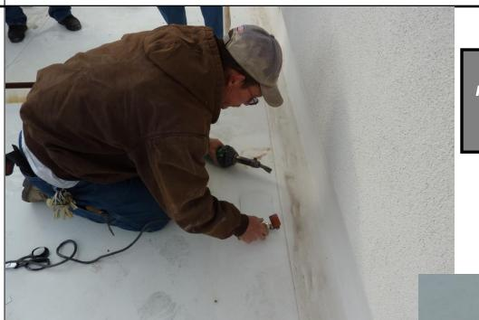
While there were no heat related failures, all attempts to heat weld/patch the roof were unsuccessful.
