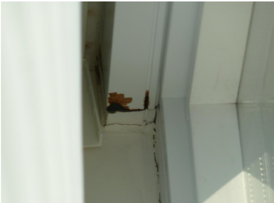
Figure 27. Interior stains from melting bitumen
