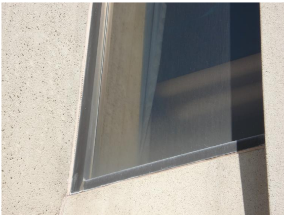
Figure 21. Sealant joint width too narrow to handle shear in sealant
