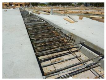
Figure 4: Post-tensioned reinforced concrete slab under construction Also common in steel structures is steel pan deck, with mild steel reinforced concrete. Prior to the adoption of reinforced concrete, the 2-way flat plate and one-way slab over beam systems were common however, not used as much anymore.
