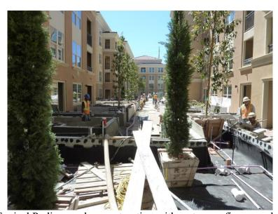
Figure 2: Typical Podium under construction with waterproofing complete inside of planters. Due to the heavy construction traffic, waterproofing membrane is phased and installed last, before the wearing course.
