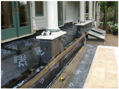
Figure 8: Combination self-adhered modified bitumen membrane with fluid applied waterproofing
