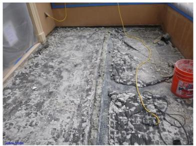
Figure 23: On this wood framed balcony deck, the drain mat was discontinuous down the center of the deck. This resulted in water not properly flowing and ponding on the upslope side of the discontinuity.
