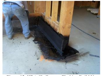
Figure 12: HRA Challenge – Flashing Build Up
