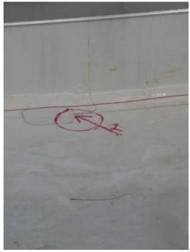
Figure 19: Pinhole leak discovered using EFVM
