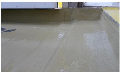
Figure 10: Asphalt modified polyurethane
