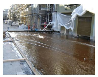
Figure 20: ASTM D5957 – Standing Water Testing
