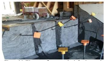
Figure 14: Waterproofing around reinforcing steel
