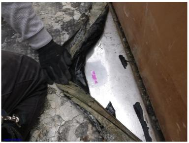
Figure 27: Adhesion failure of cold fluid applied membrane to stainless steel flashing due to lack of proper priming and prep work.
