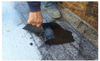
Figure 11: Adhesion of membrane with sheet neoprene
