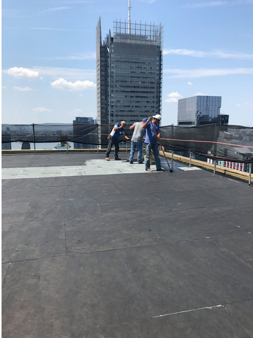
Figure 19 - Primer Being Applied
