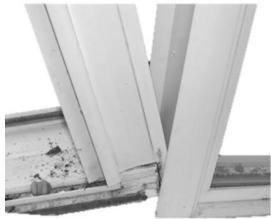
Figure 2A – Common Window Failures
