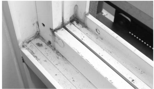
Figure 4A – Coped Mullion Joint Failure
