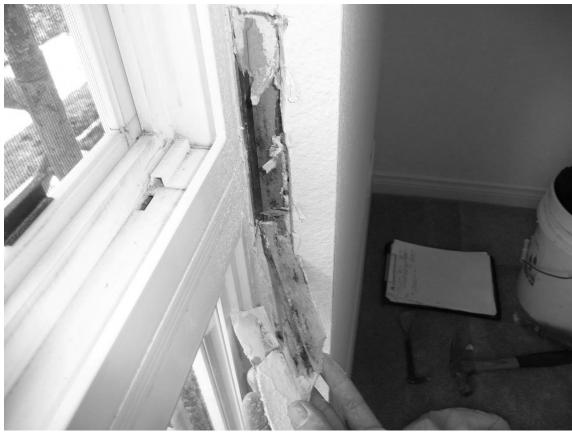
Figure 3A – Vertical Mullion Failure
