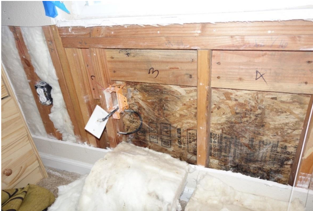
Figure 8: Uniform Damage Behind Fiber Cement Siding
