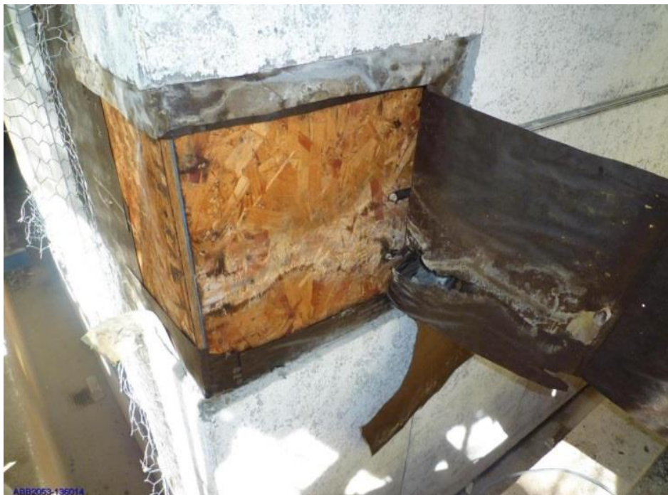
Figure 9B: Control Joint Impedes Water Drainage
