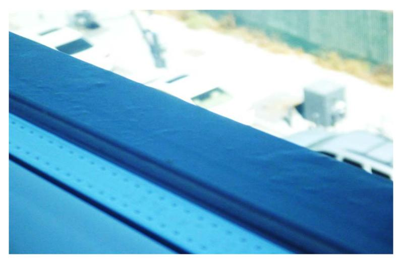
Coating is bubbling on window frames
