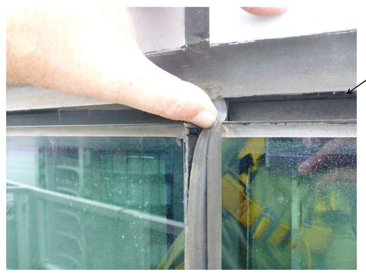
If the ends of the sealant joints are not closed, water is able to infiltrate on top of the primary seal
