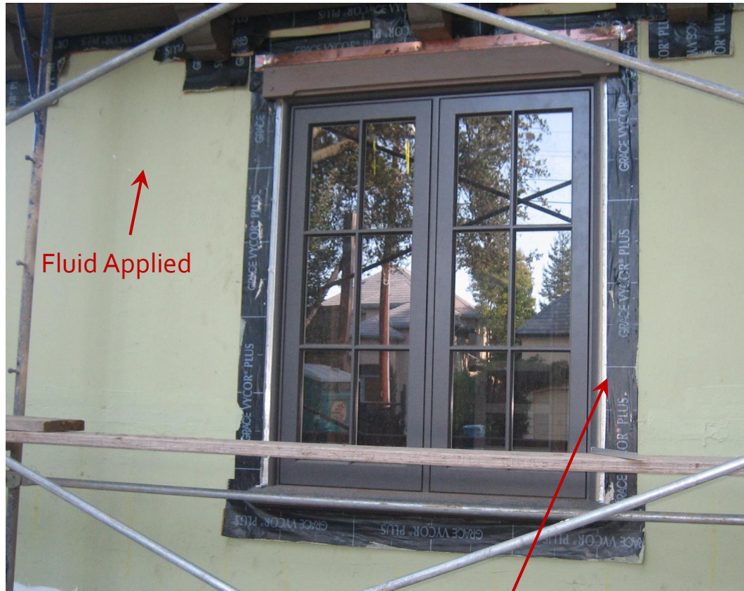
Window sealed with Flexible Flashings
