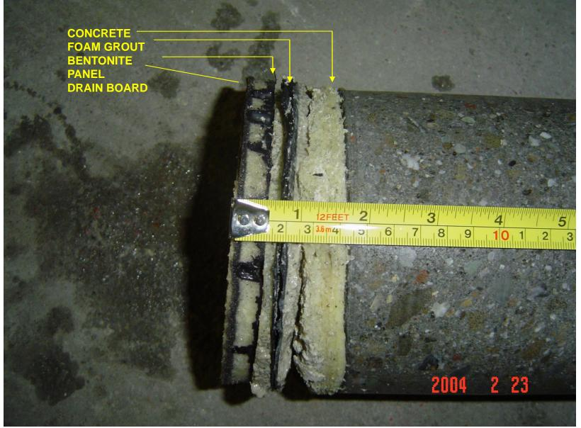
Voids were present on both sides of the retaining wall and ranged from 1" thick to up to 4" thick.
