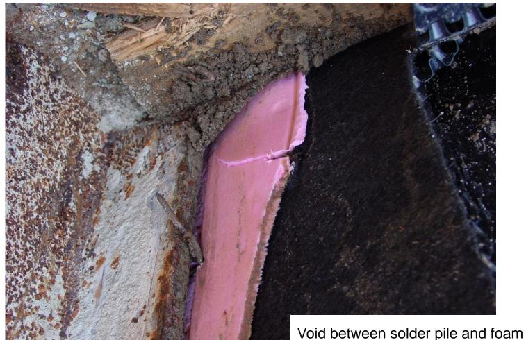
protection board was also evident and may have contributed to the failure of the bentonite waterproofing system.
