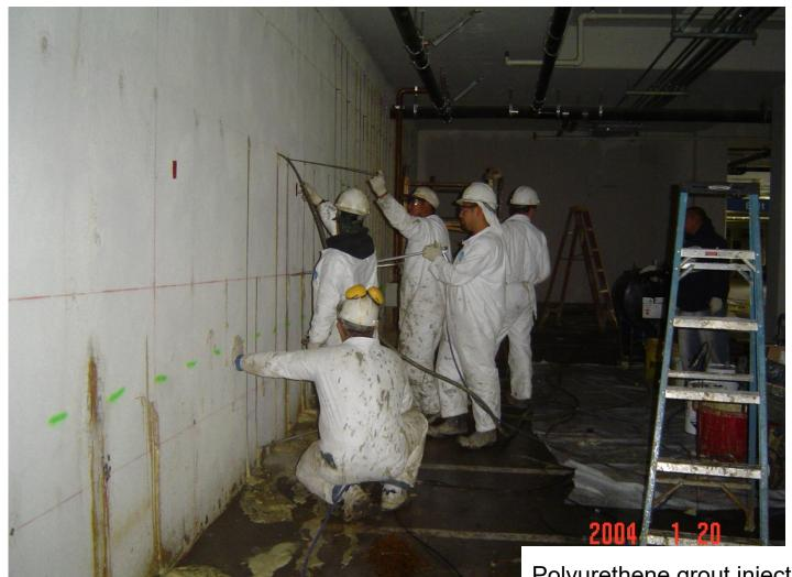
Polyurethene grout injection 2' on center at a cost of \$35/SF
