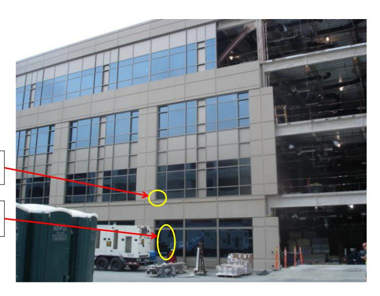
Leak observed on the 2<sup>nd</sup> floor after the first spray test at the GFRC panel
