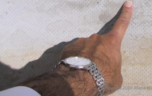
**Erosion of membrane due** to water had deteriorated membrane, scrim is visible.
