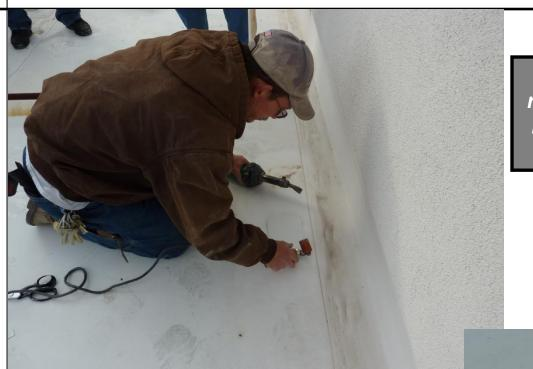
While there were no heat related failures, all attempts to heat weld/patch the roof were unsuccessful.
