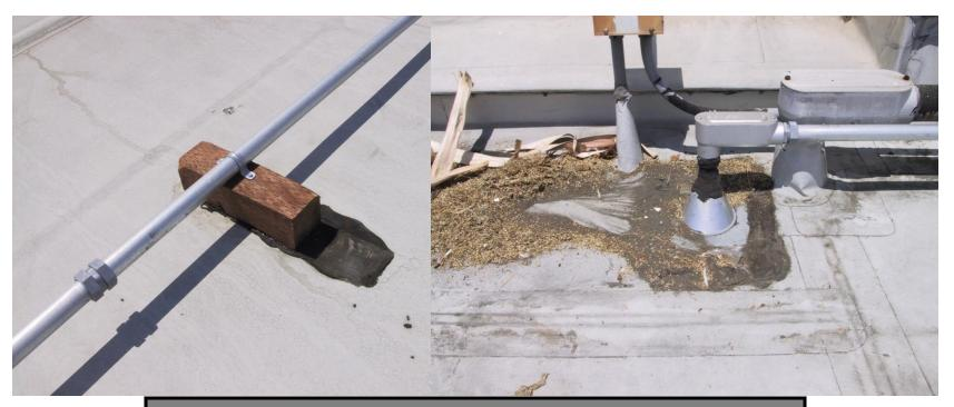
New electrical pipe added, pipe jack set in mastic (not properly flashed with single ply) and wood block set in mastic (incompatible with PVC).
