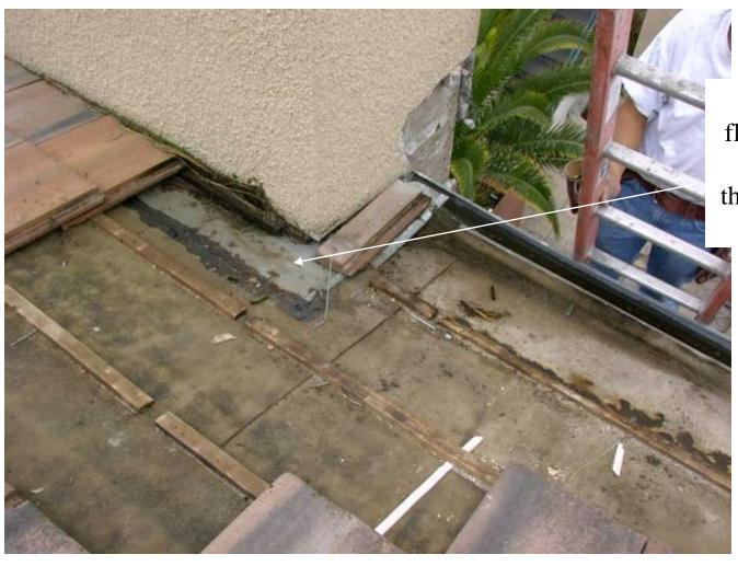
Roof to wall flashing installed as an after thought, on top of felts
