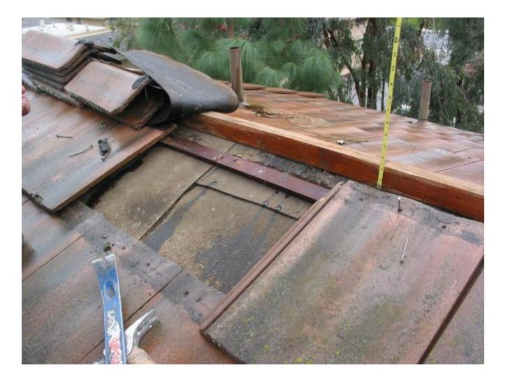
Water penetration but this was not the primary source of leak in unit below. Improper membrane was utilized as wind block. 30lb felt was used instead of 9" pressure sensitive adhesive membrane recommended by material manufacturer.
