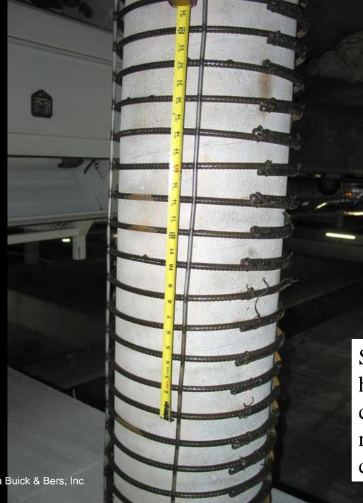
Some of the heavily stressed columns were reinforced with concrete and rebar
