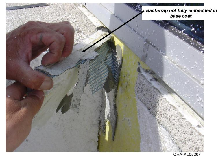
Test Cut #3– East Elevation – 4<sup>th</sup> floor line EIFS Bullnose. Required by Dryvit
